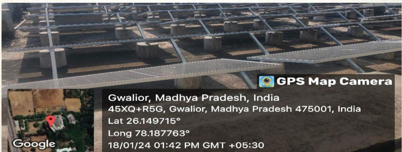
Photos of Solar panels on the roofs of JC Bose Block building
